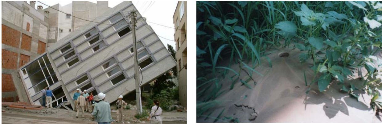
Figure 2: Examples of liquefaction in Adapazari
