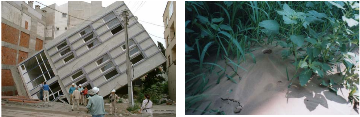
Figure 2: Examples of liquefaction in Adapazari
